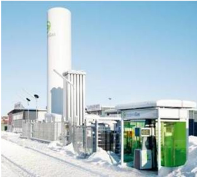
L-CNG filling station in Göteborg (Sweden)
